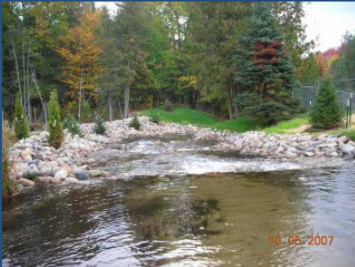
Example- Natural Rock Riffle Structure in Grand Traverse County.
